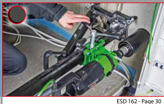
Drilling in hard materials
