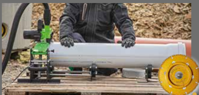
Align the pipe exactly horizontally and vertically to the saw blade
