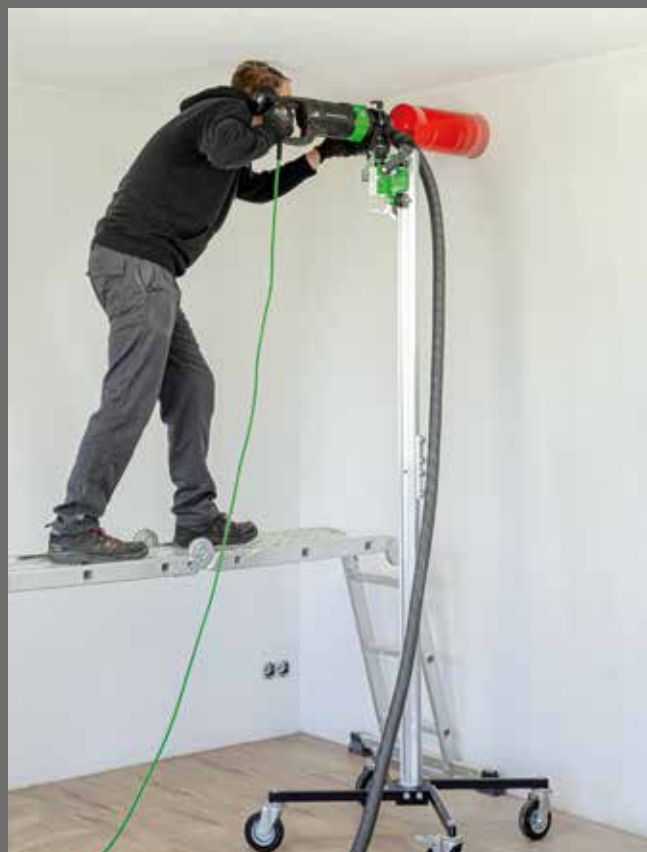
Ventilation holes up to 2.30 m height with column extension
